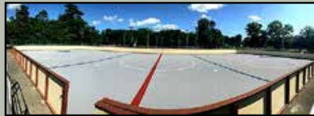
The Hockey Court at Michael Debbi Park received much needed repairs
