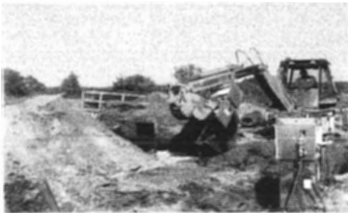
Pulled diesel tank
